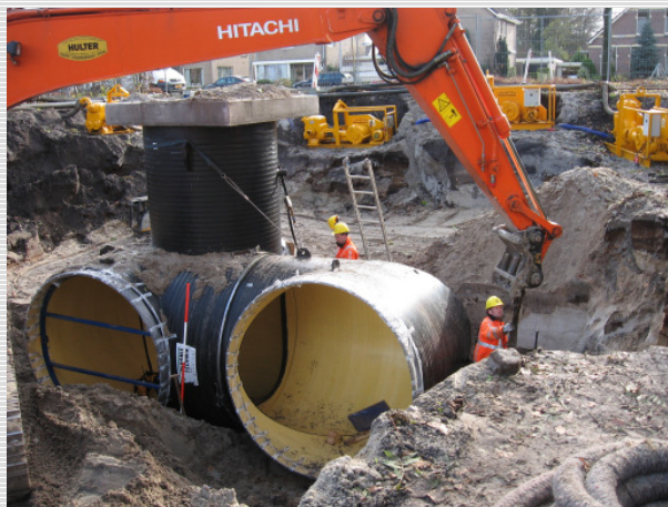
Pict: 1: Special construction ND 2300 with pump manhole ND 1800
