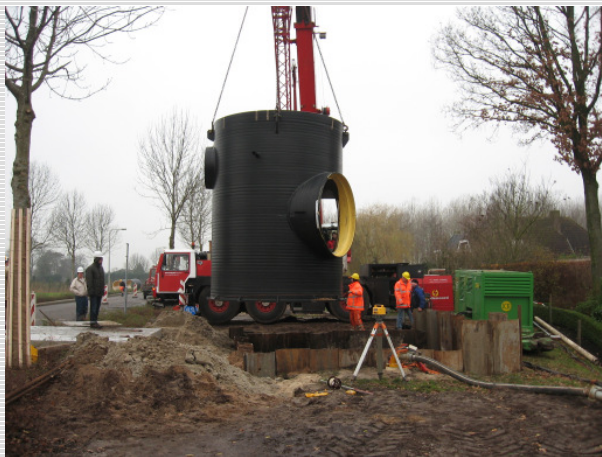
Pict. 3: Setting of overflow-/pump manhole ND 3000
