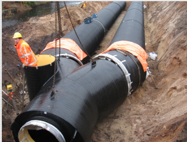
Pict. 4: Assembly of inlet structure ND 1800 with integrated inspection chamber ND 1000
