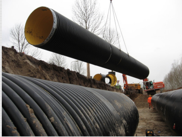
Pict. 2: Installation of 18m length PKS-pipe ND 1800
