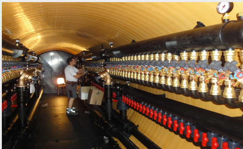
Picture 5: Factory-provided pre-assembly with all essential stop and regulating valves
