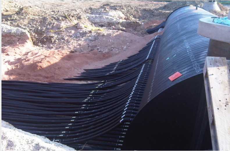
Picture 6: on-site connection of the probes to the manhole
