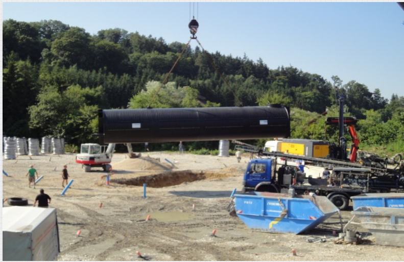
Picture 4: Location of manhole into the building pit
