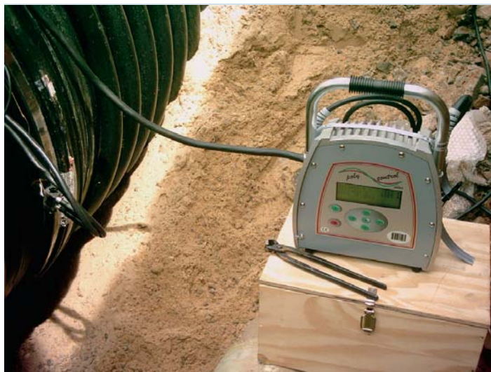
Bild 5: Heizwendelschweißen an einem Wickelrohr d 1.800 mm Fig. 5: Sleeve welding with an incorporated electric heating element on a wound pipe, d 1,800 mm
