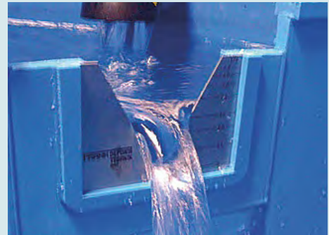
Measuring weir to determine the capacity in a spring water collection chamber
