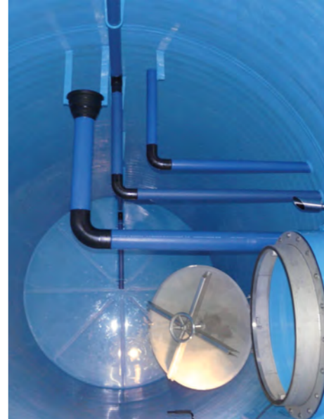
Water reservoirs arranged in parallel with central access to the controls and instruments chamber.
