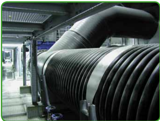
Fig. 164 - PKS® T-piece with elbow
