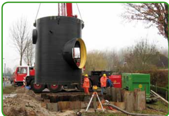
Fig. 170 - Installation of DN 3000 overflow/pump shaft
