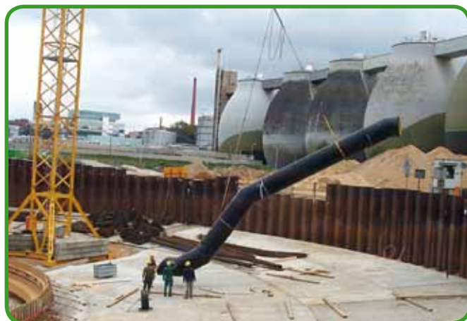
Fig. 73 - Unloading and positioning of PKS® DN 3000 pipe
