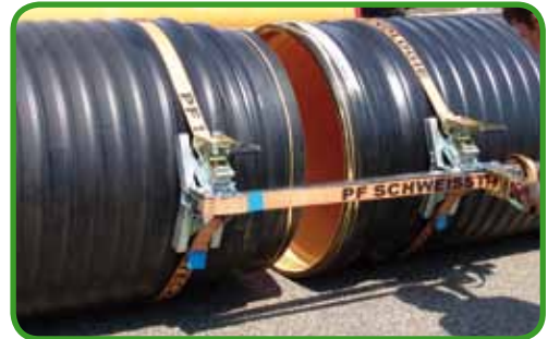
Fig. 101 - Pulling the pipes together
