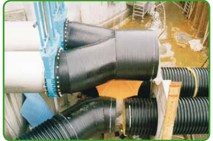
Fig. 147 - PKS® Y-piece, flange-mounted
