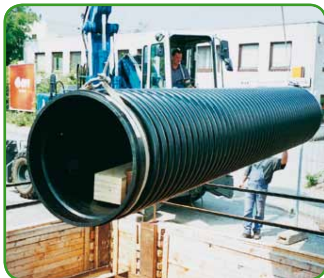
Fig. 54 - PKS® pipe with electrically conductive inside layer
