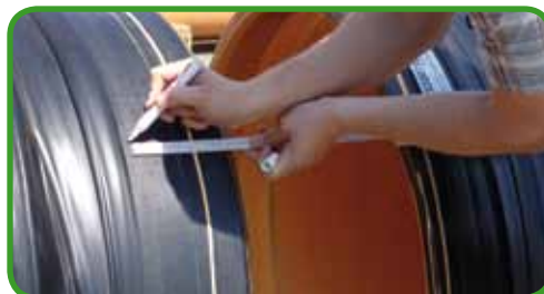
Fig. 100 - Marking the insertion depth
