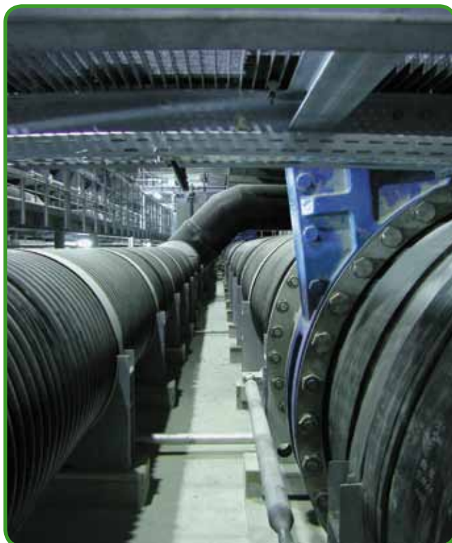
Fig. 165 - PKS® pipe flange connections
