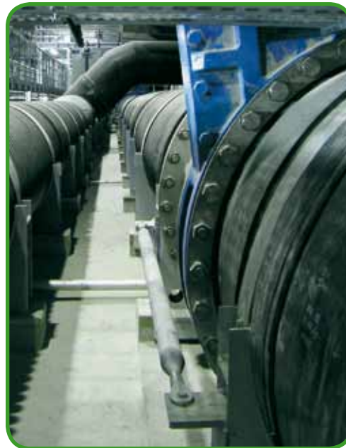
Fig. 134 - Flange connections in sewage treatment plant
