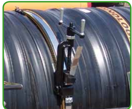
Fig. 102 - Tightening of tension bands
