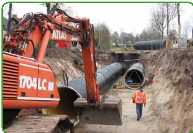
Fig. 167 - Installation of PKS® pipes
