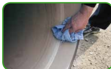
Fig. 130 - Cleaning the socket
