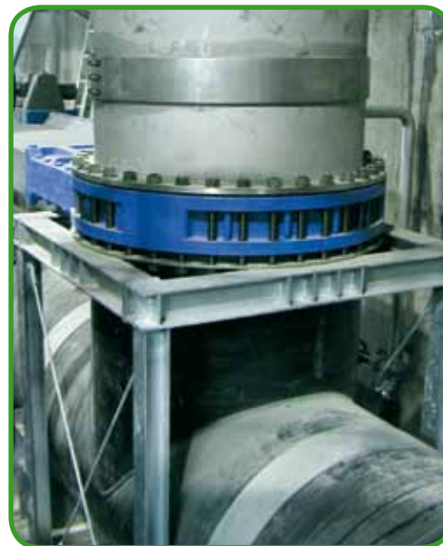
Fig. 135 - Flange connection to PKS® pipe
