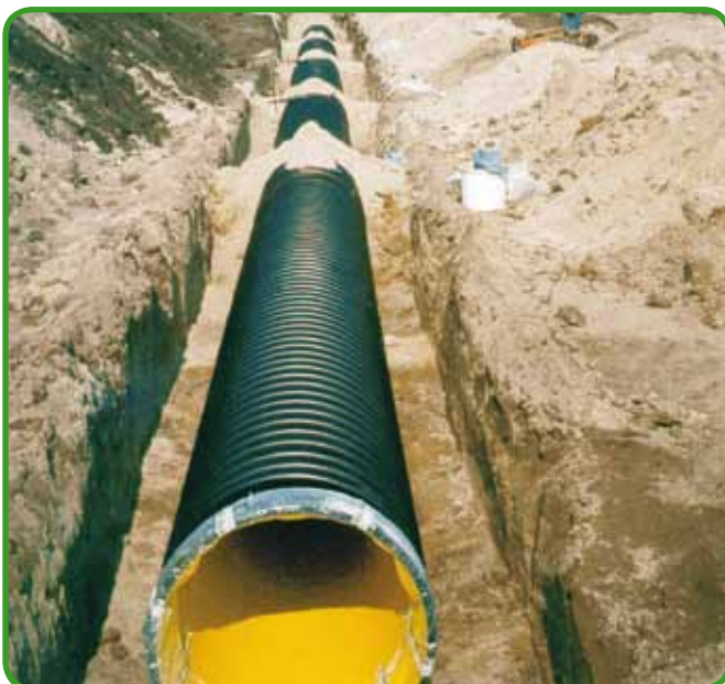
Fig. 65 - PKS® sewage pipe installed in pipe trench
