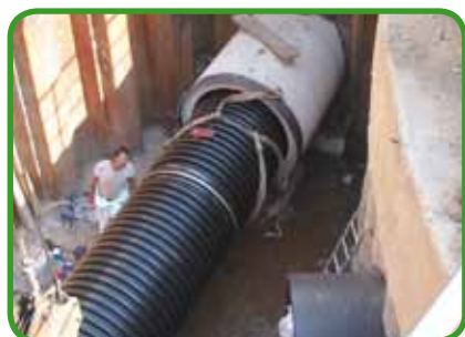
Fig. 86 - Short pipe relining
