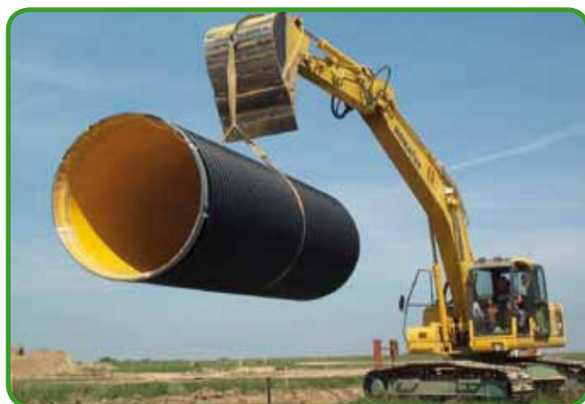
Fig. 72 - Unloading and installation of PKS® DN 1800 pipe
