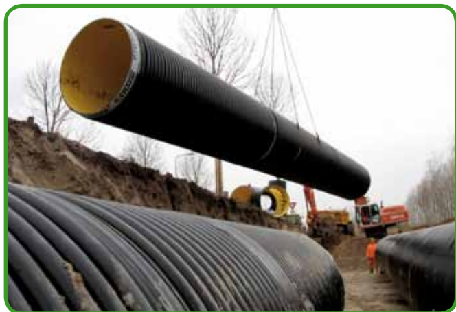
Fig. 169 - Laying of PKS® pipe DN 1800, in pre-welded sections of 18 m
