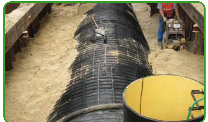
Fig. 77 - Compacting of side bedding
