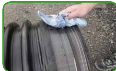
Fig. 128 - Cleaning the spigot end
