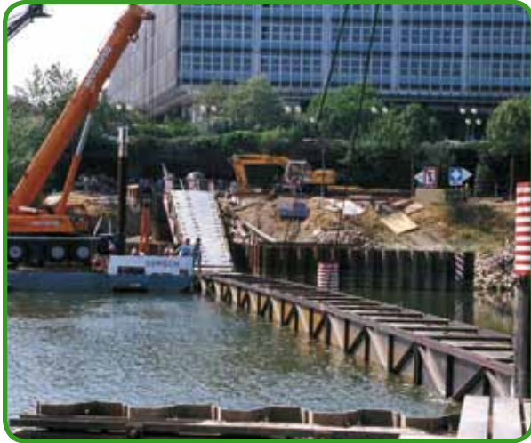
Fig. 158 - Neckar under-river pipeline section is being lowered to the bottom of the river bed
