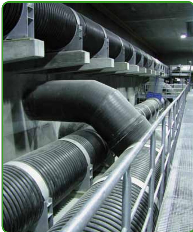
Fig. 163 - Supports/clamps for r PKS® pipes
