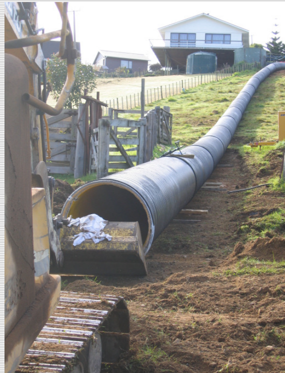
Picture 2: Preparation for installation
