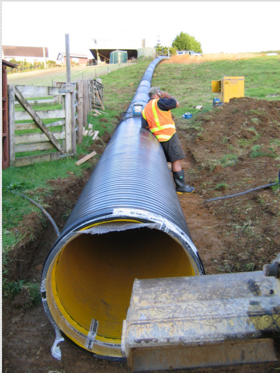
Picture 1: DN 800 SQ1 34-10 section of spiral pipe SQ-Profile/New Zealand
