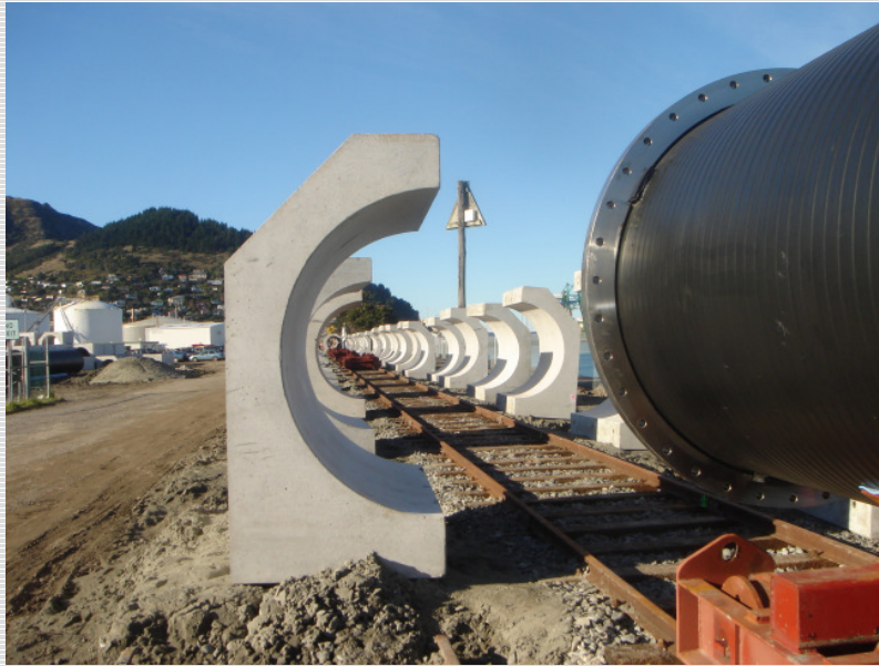
Picture 4: Installation of concrete anchors
