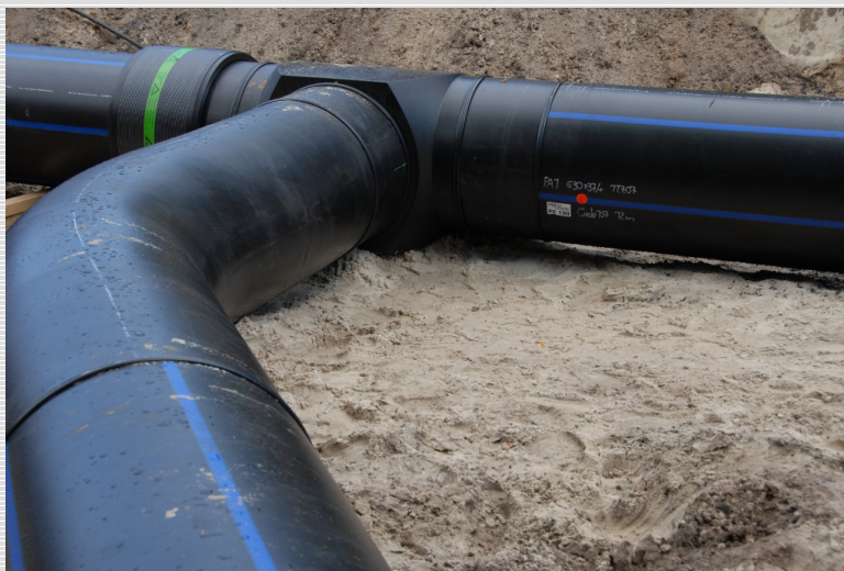
Abb. 3: Complete installed and welded PE 100 Tee 630/400 mm
