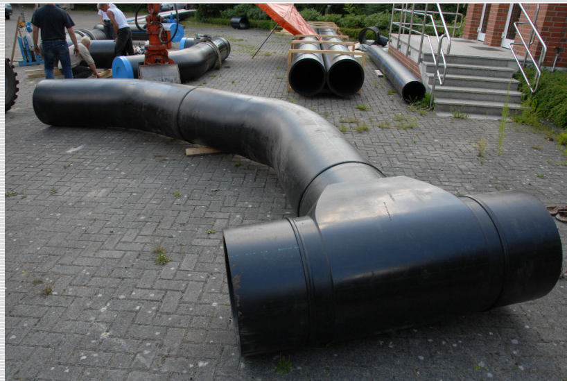
Abb. 1: Preparation of PE 100 fittings d 630 mm
