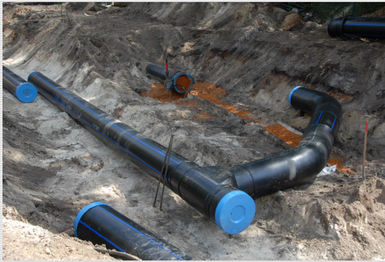
Abb. 2: Installation in pipe trench
