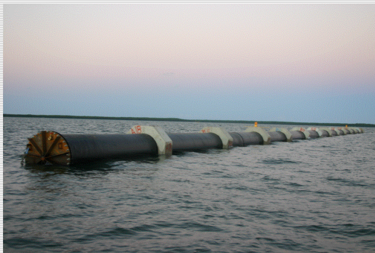
Picture 2: Pipe with concrete anchors before submerging
