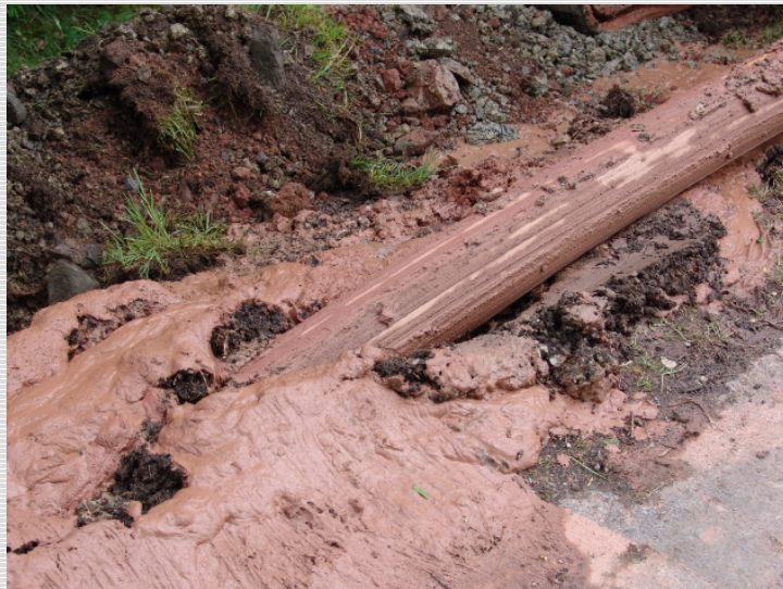
Abb. 3: Target of HDD. The pipe come to light.
