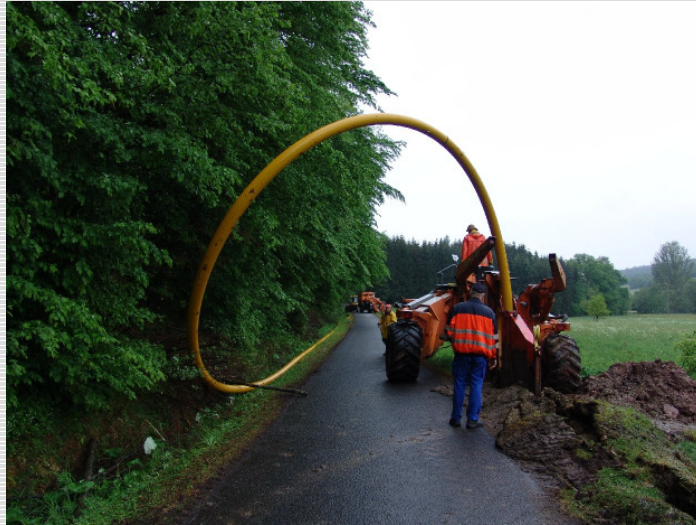
Abb. 2: Plowing of Surline II - pipeline at the roadside
