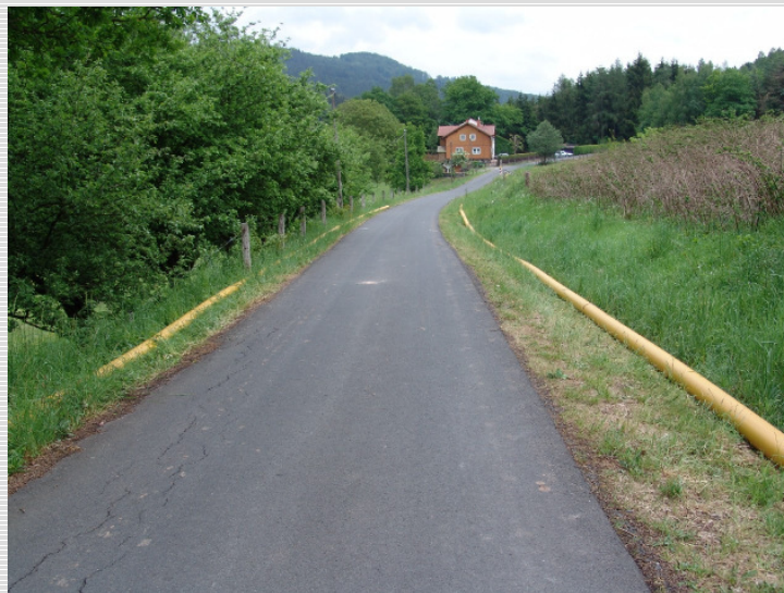
Abb. 1: Countryside of Rhön, with the prepared pipes
