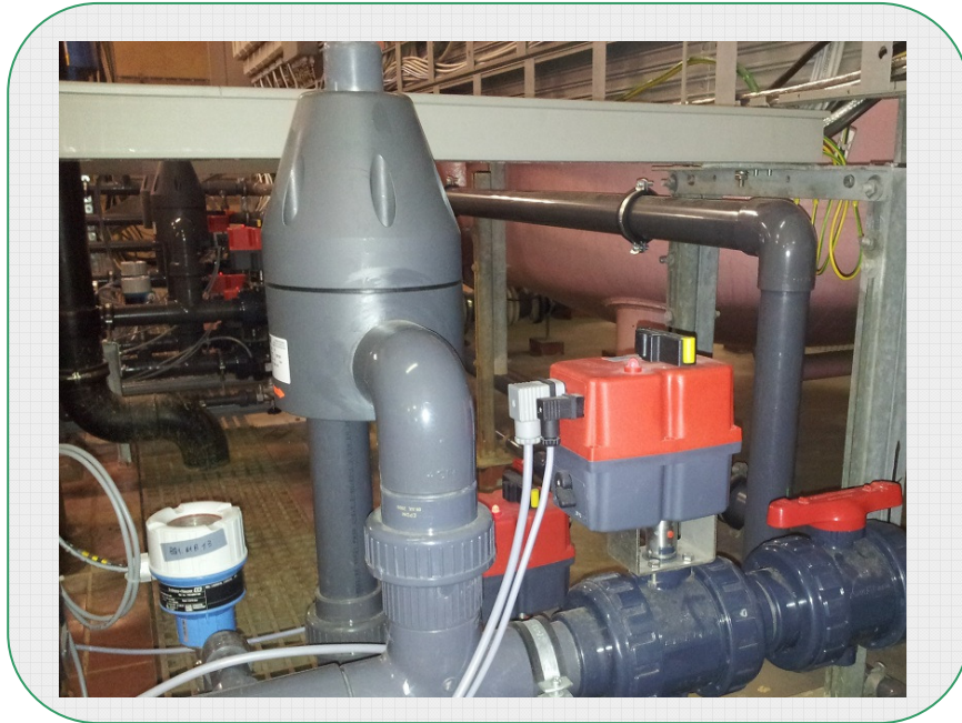
Pic. 4 pressure retaining valve as system protection
