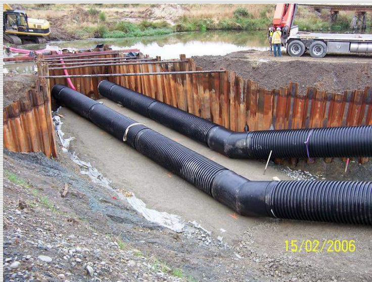
Picture 2: River crossing realized with PKS-system
