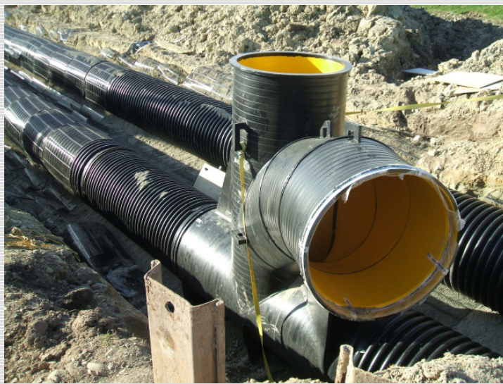
Picture 3: ID 1200 mm pipe with riser and shaft
