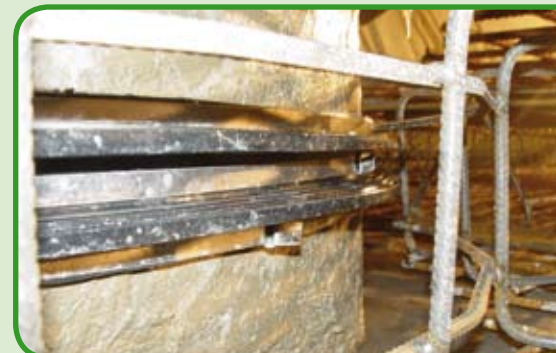
Puddle flange mounted on manhole
