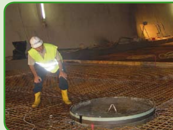
Manhole before pouring the waterproof concrete
