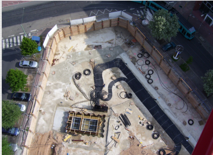
Picture 2: View from a crane onto the geothermal pipes
