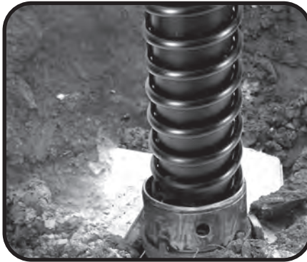
Insertion of VTP® in the borehole with hollow stem auger
