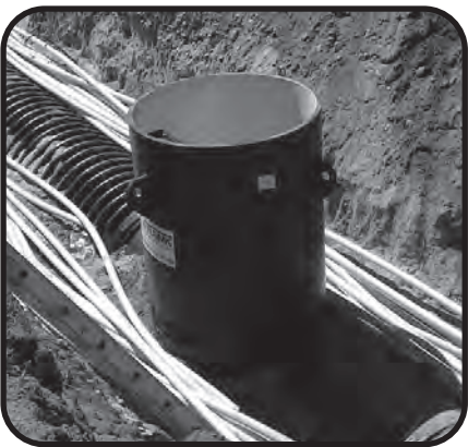
Parallel installation of connection pipe close to Chamber manifold
