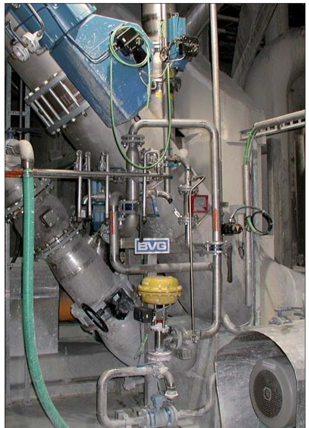
Bild 9: Kalkmilch-Regelventil DN 65 in der Papierindustrie Fig. 9: Milk of lime control valve DN 65 for paper industry
