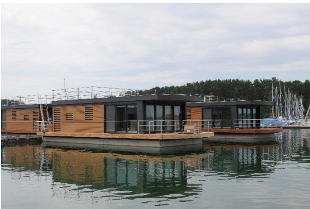
Die Floating Houses am Brombachsee
